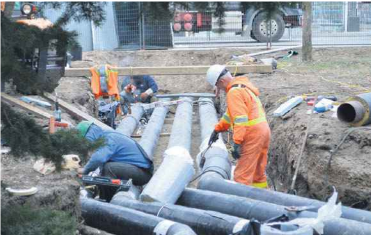
Workers install pipes at Guelph’s Sleeman Centre, which will be part of North America’s first city-wide district energy network. In addition to bringing massive savings in fuel, equipment and maintenance costs, this initiative will lead to a much smaller environmental footprint. SUPPLIED
