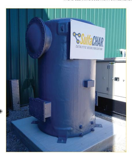
Distributed by CharTech Solutions, **SulfaCHAR**<sup>TM</sup> is a cost-effective, convenient system with two options: a High-Capacity and a Zero-Waste. Both options are targeted gas cleaning solutions for hydrogen sulfide in renewable natural gas. The **SulfaCHAR**<sup>TM</sup> system efficiently filters  $H_2S$  out, greatly reducing maintenance costs.
