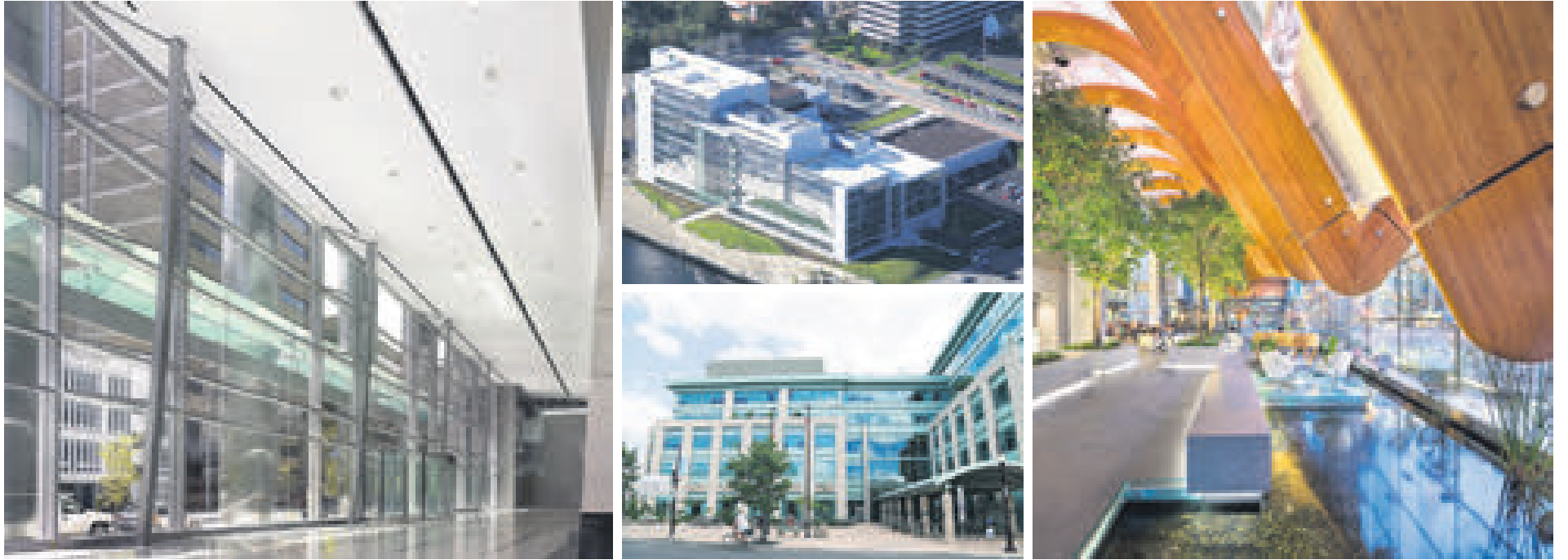
The LEED (Leadership in Energy and Environmental Design) program has seen enormous uptake in Canada over the last decade. Among the notable LEED Platinum-certified buildings across the country are (clockwise from left) TELUS Garden in Vancouver, B.C., Robinson Place in Peterborough, Ontario, Centennial Place in Calgary, Alberta, and Nova Scotia Power Headquarters in Halifax, Nova Scotia. For more information about the buildings' green features, see globeandmail.com/adv/sustainablebuilding . SUPPLIED
