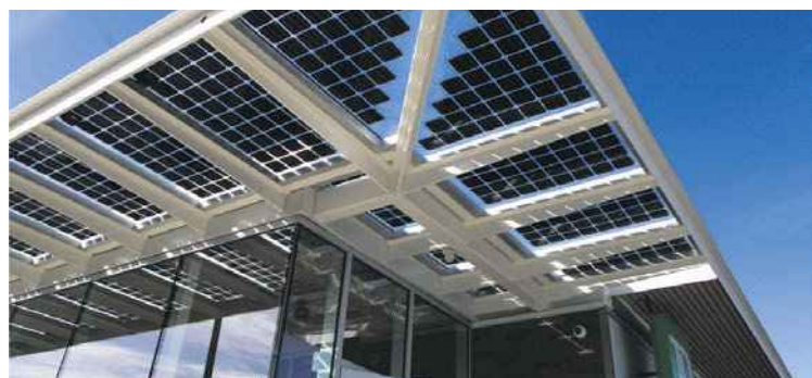
TD Bank Group's sustainable energy efficient design (SEED) branch in Mississauga is 38 per cent more energy efficient than a traditional branch. SUPPLIED
